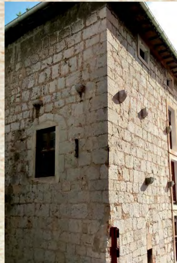
The tower of Sasiola. Tour Sasiola.
